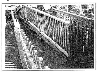
(Zone 7 - Family Flyer) A child could crawl through - under exit ramp and be exposed to the Family Flyer track area.
