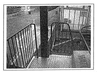
(Zone 4 – Crazy Mouse) On 8/29/07 at 11:15 AM – top of the crowd control fence has been welded within 4 inches from roof support column. It was painted before opening.
